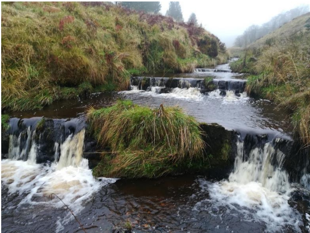
Figure B-4 Bedrock steps in River Nethan
