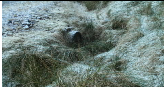
Existing 450Ø HDPE pipe inlet
