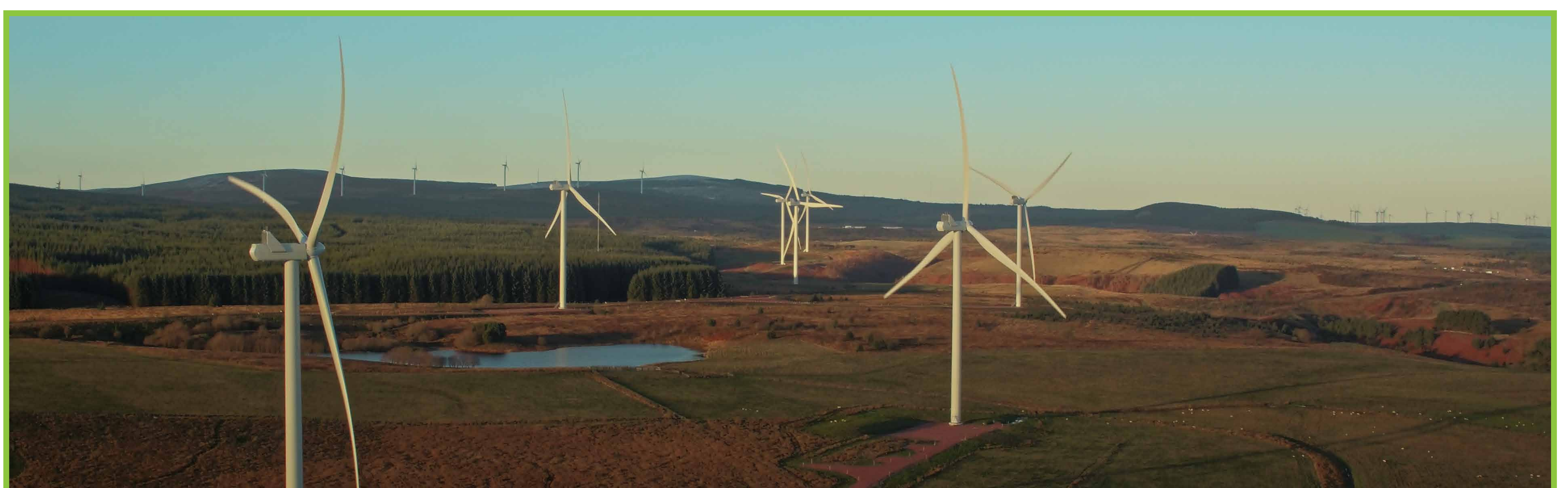
Picture looking west through Douglas West Wind Farm within Hagshaw Energy Cluster
