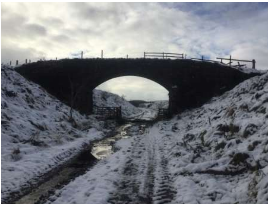
Photograph 2 Former Railway Bridge at NS 82631 32103
