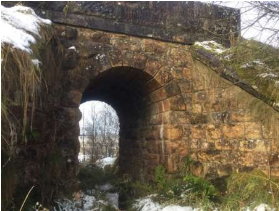
Photograph 1 Former Railway Bridge at NS 83 083 32593
