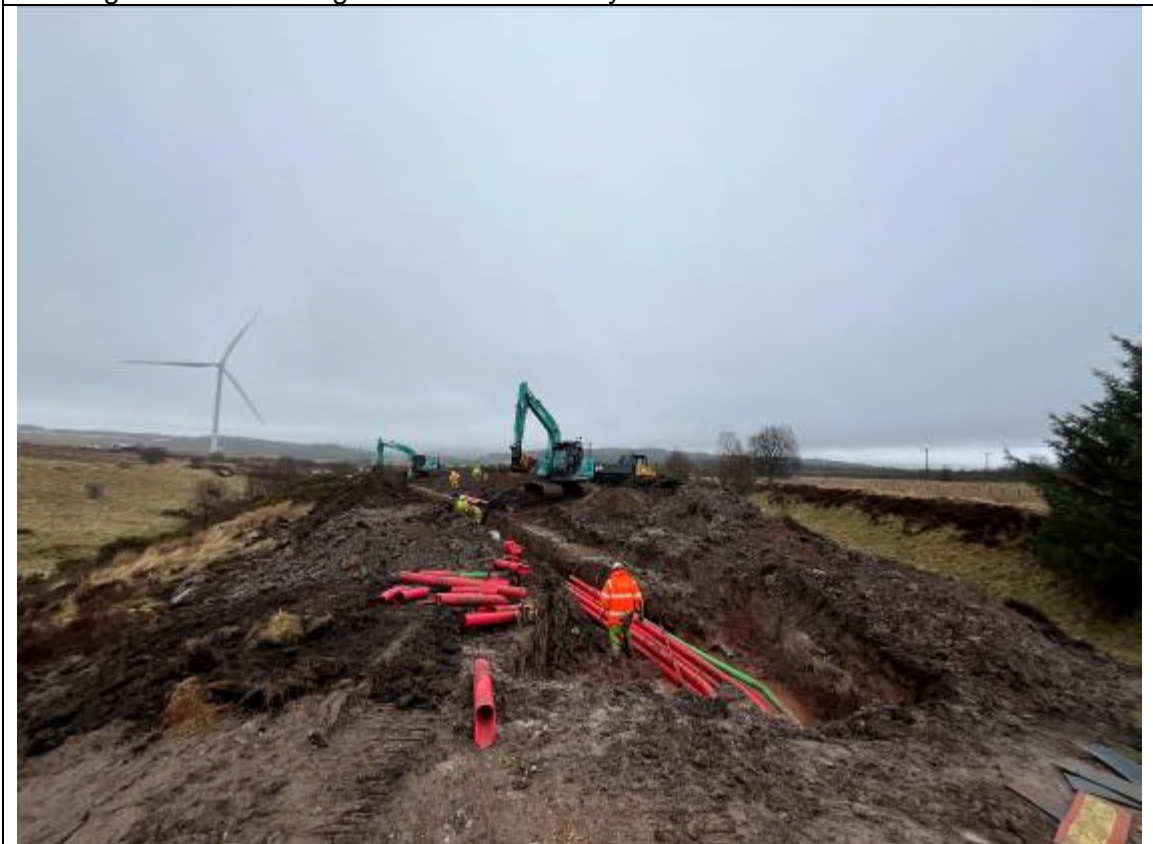
Area adjacent to southern boundary of site. Current works ongoing to lay electricity cables.
